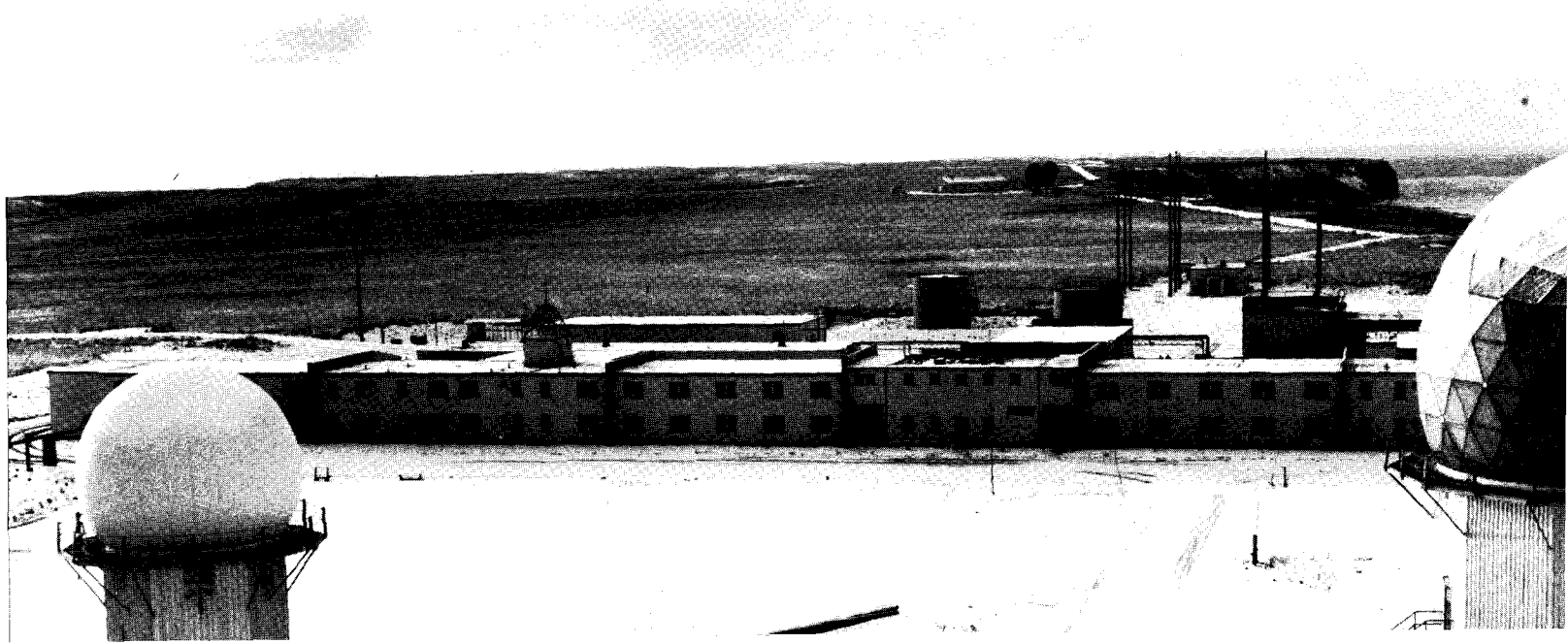
(below) Radar domes, scattered buildings, tundra, a vast view of the sea . . . this is Middleton.
